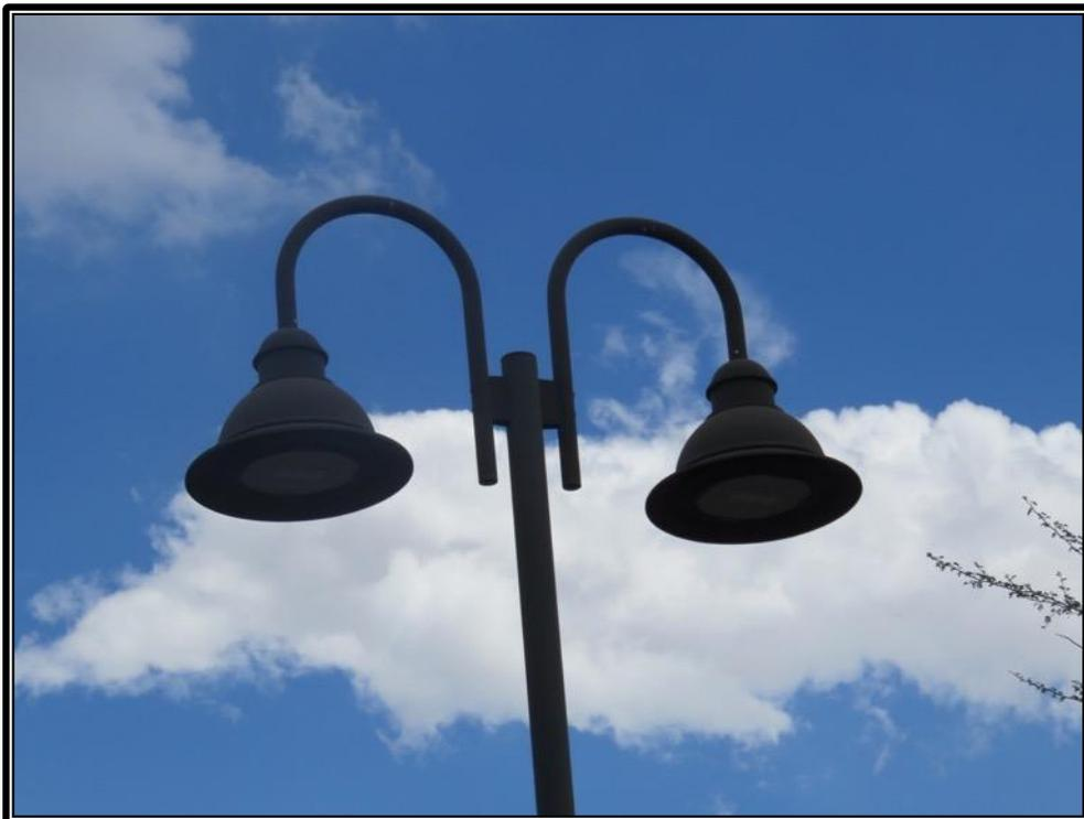
*Pendant-style metal halide lights that were replaced with 2700K LED lamps*
