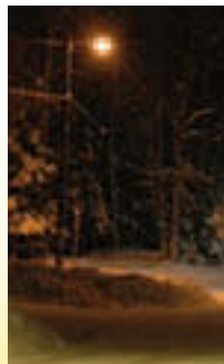
High Pressure Sodium Lights
